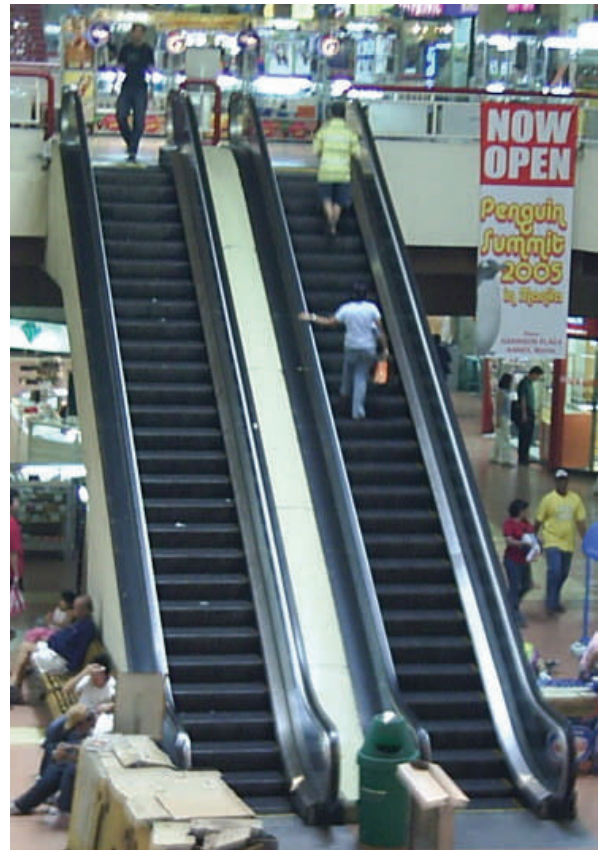
The Up-Bound Escalator on the Right was Fitted with EnviroStart
