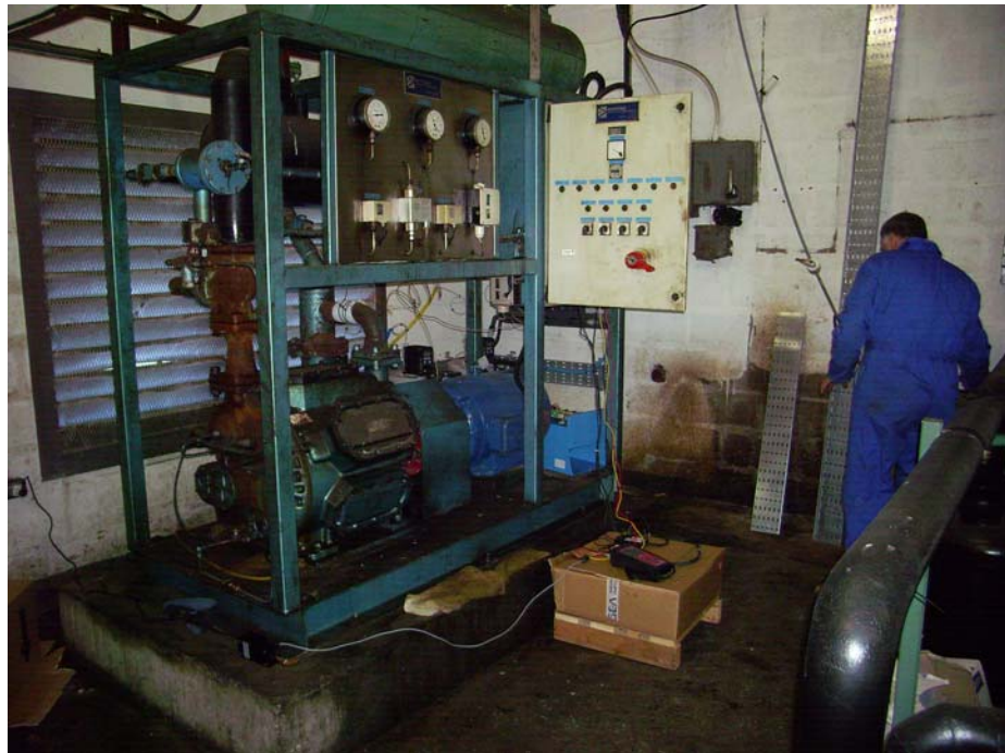
Figure 4: Installation/commissioning of 55 kW MEC unit
