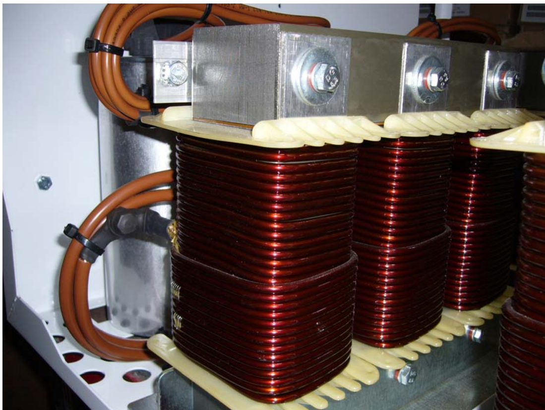
A Typical Inductive Reactor Used for Harmonic Filtering in a Detuned EnviroVAR Cabinet
