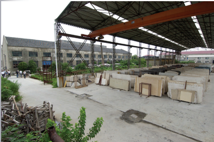
Ding Li Slab Storage Facility Adjacent to the Cutting Room
